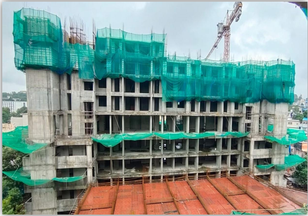
D WING – 4 TH RESI. SLAB CASTING IN PROGRESS
