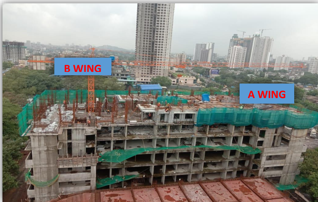
A & B WING – ALU. FORM WIP FOR 3 RD RESI. SLAB
