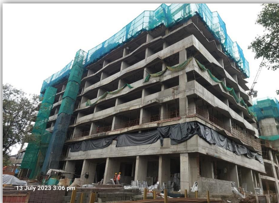
B WING – ALU. FORMWORK IN PROGRESS FOR 2 ND TOP SLAB
