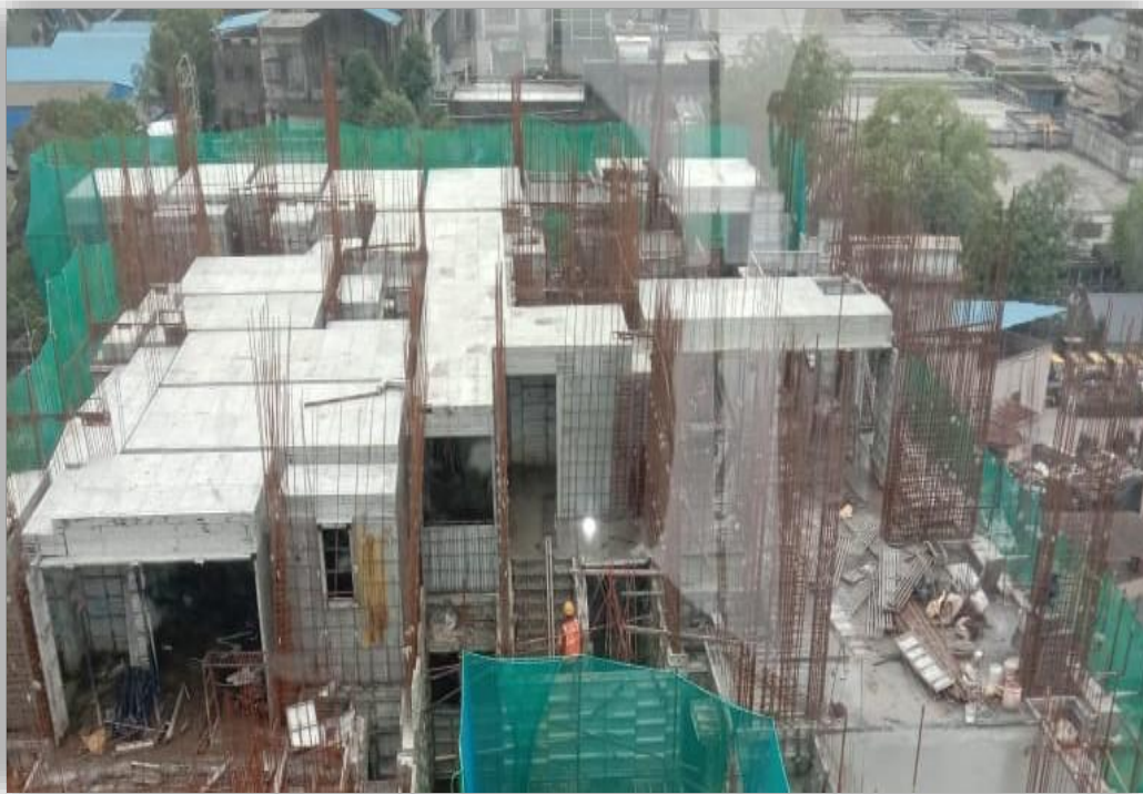
Wing C : ALU. FORMWORK IS IN PROGRESS FOR 5 TH RESI. SLAB
